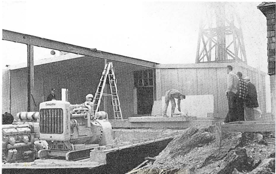
FIG. 18. Once the transmitter room had been enclosed, the station began operation.
