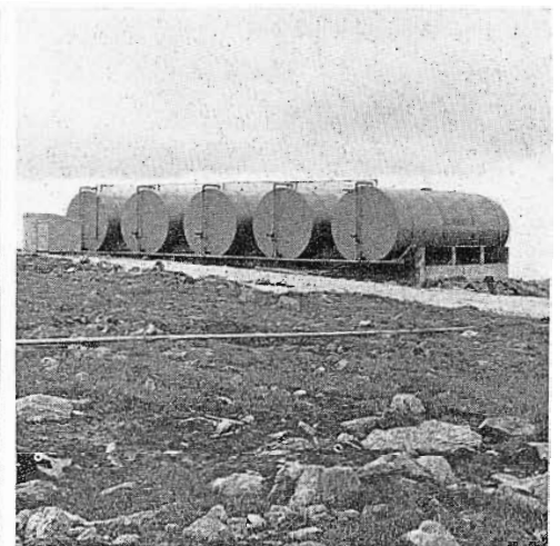
FIG. 10. WMTW's fuel is stored in five 20,000 gallon tanks. These tanks hold a full year's supply of fuel.
