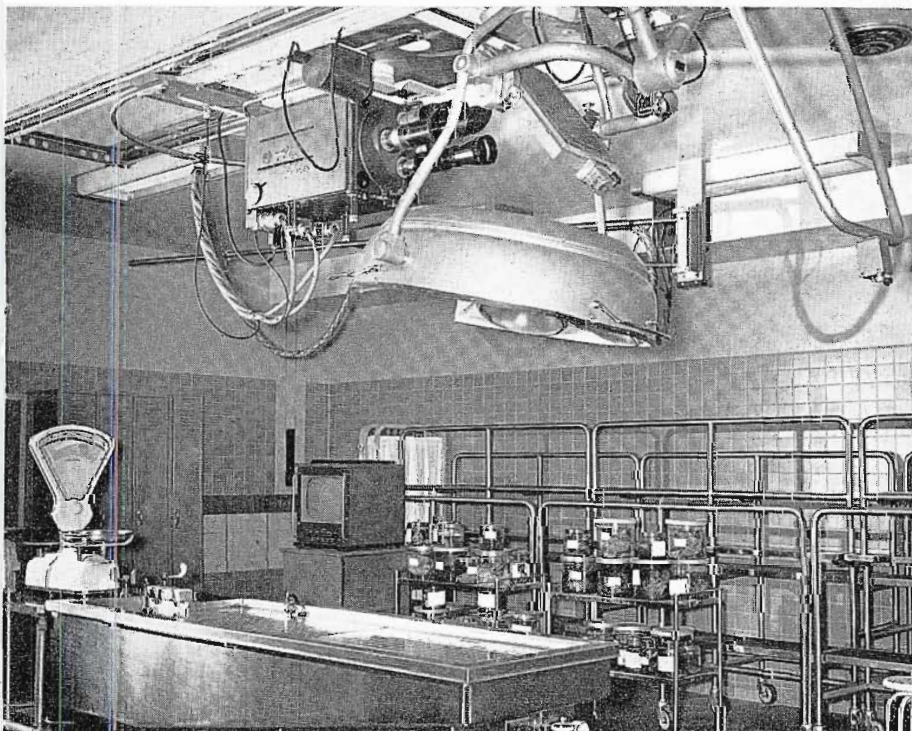
FIG. 10. Medical Color TV Camera is also used in autopsy suite to demonstrate post-mortem surgical procedures. Camera is remotely controlled.
